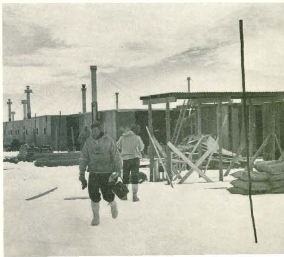
Right: The completed buildings with some of the left-over materials.
