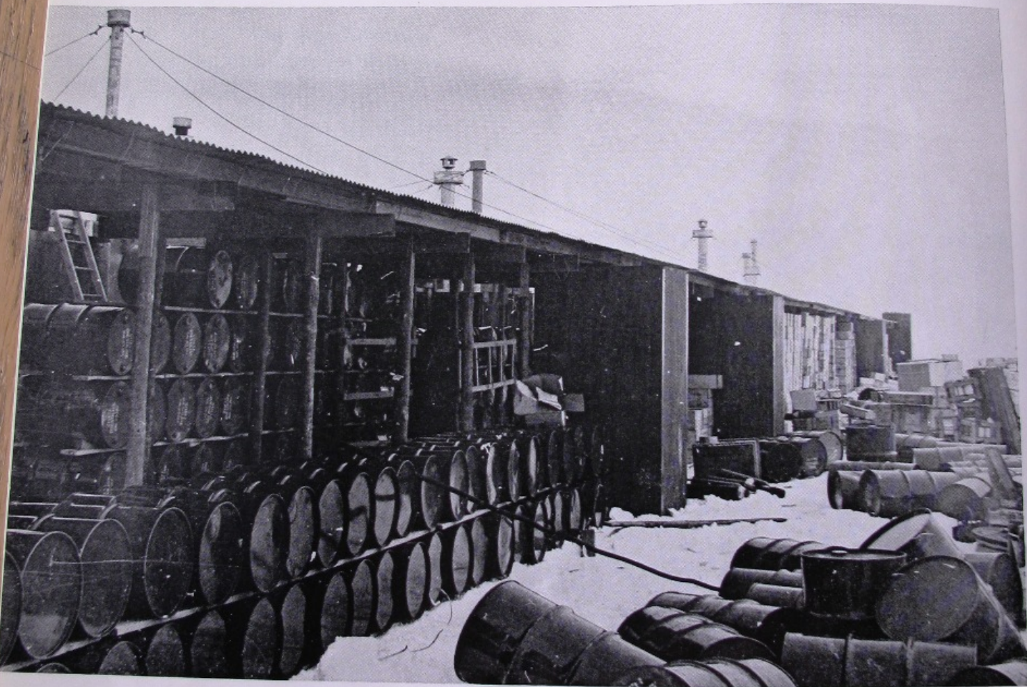
Establishing a bulk fuel supply in the south end of the snow-passage.
