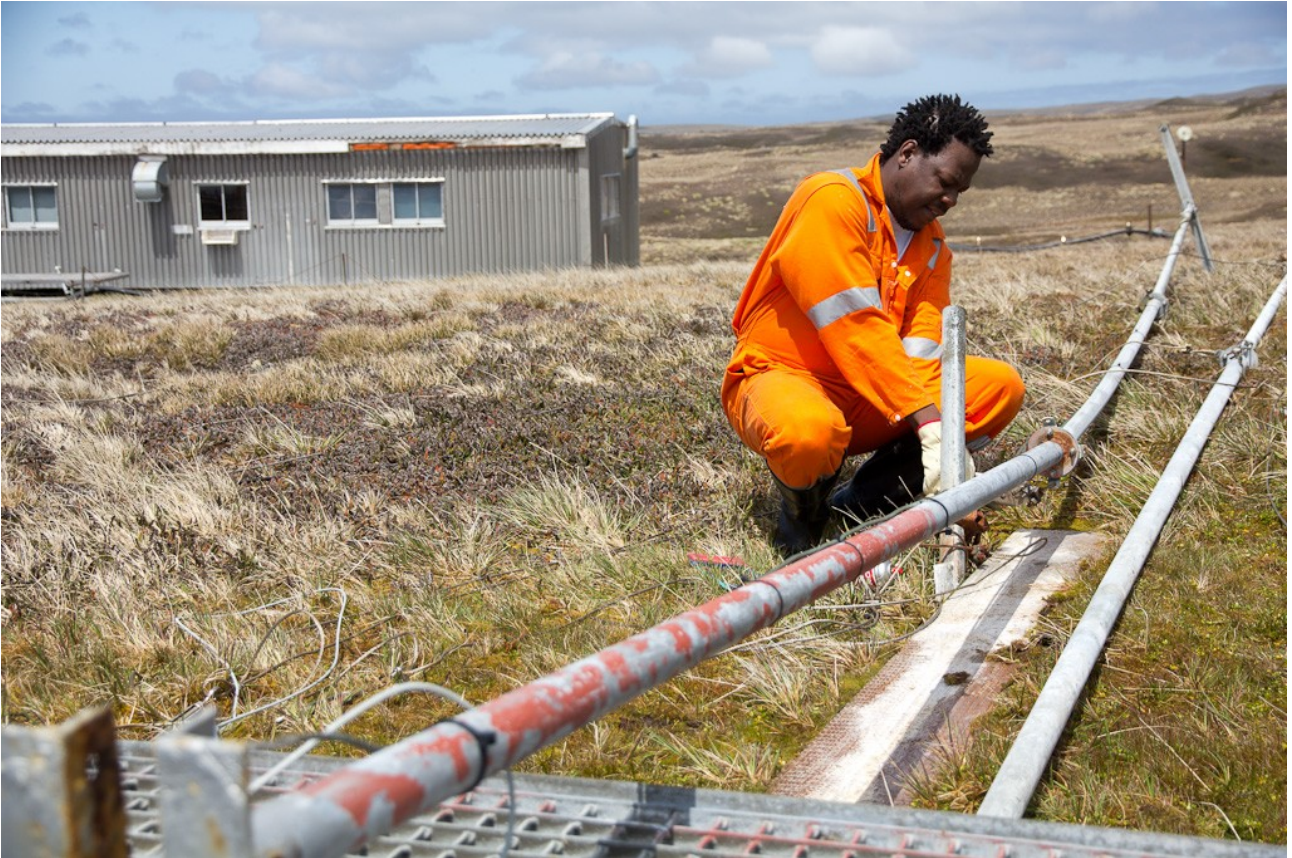
Above: Old mast on the left new mast on the right
