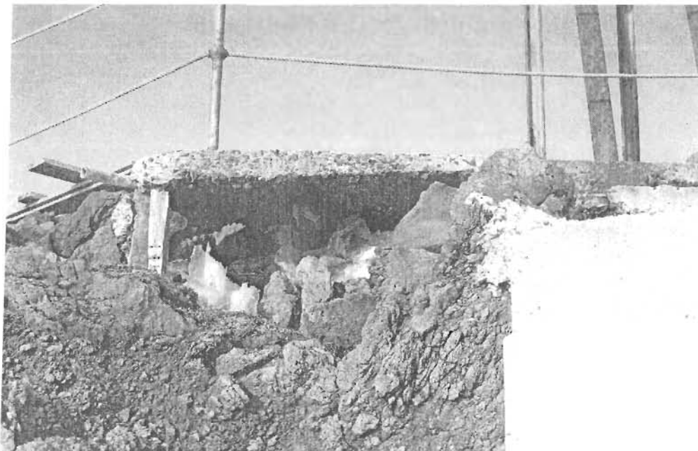
OLD BUILDING RUBBLE AND BASE WASTE USED AS 'FILLING'
