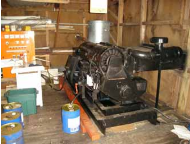
Deutz Genset which operates the Crane + supplies the whole base with electricity.
