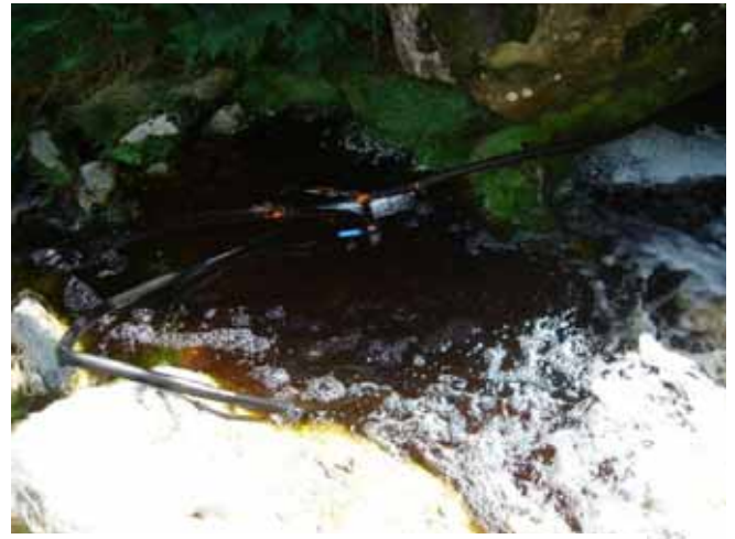
The Picture above is where we get our base water. As you can see above the PVC pipe is kinked due to heavy rain.
