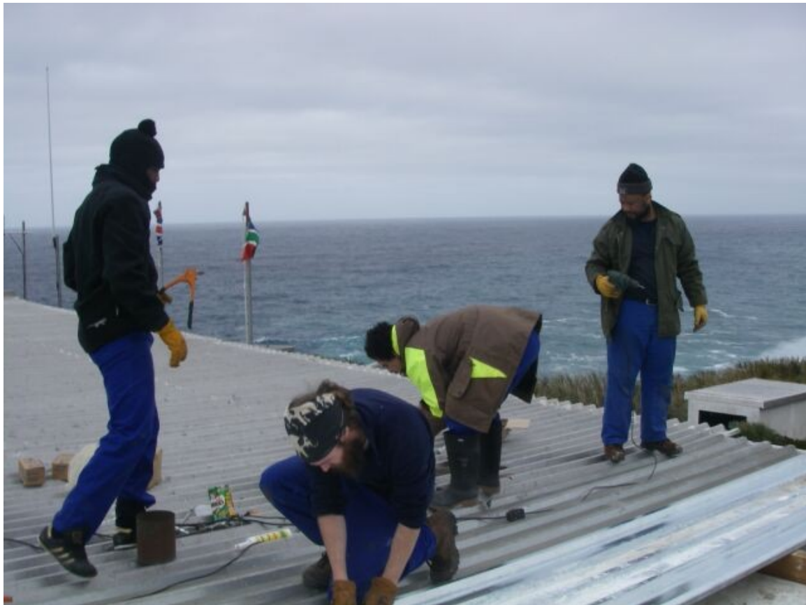
Everyone getting "stuck in" repairing the roof.
