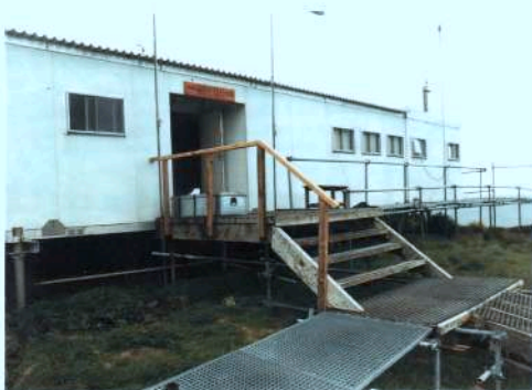
MAIN ENTRANCE TO COUGH HOUSE
