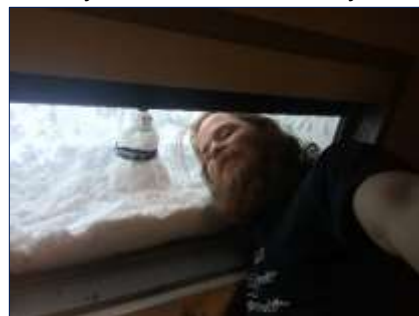
Figure 2. The window in my room was not sealed 100% and snow piled up on the inside of my window during a snow storm. So I made a snow man !
