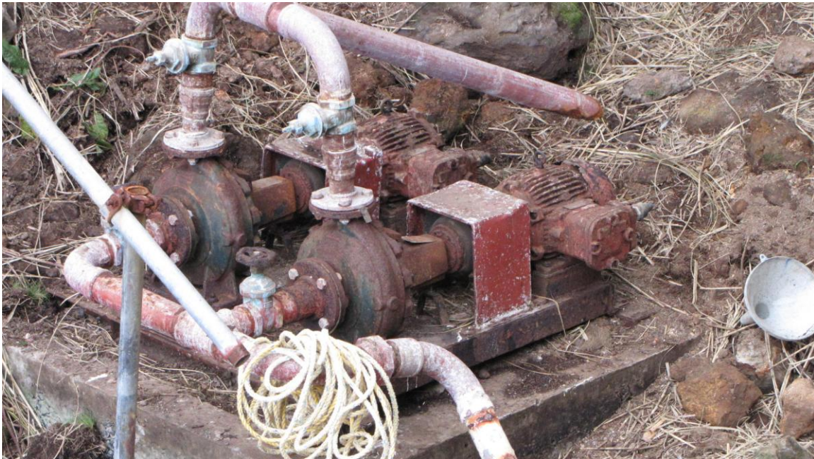
Fig. 4. Disused fuel pumps scheduled for removal in 2010
