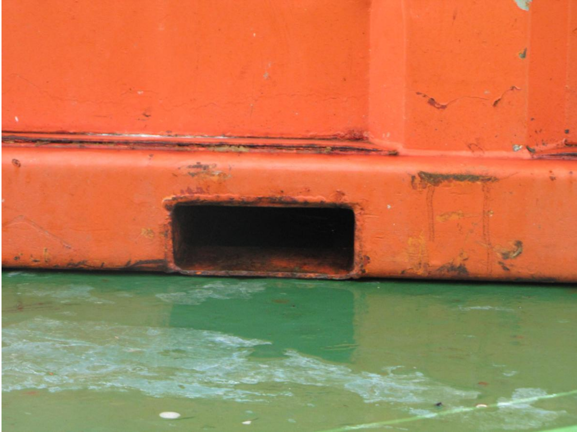
Fig.3. Fork-lift opening in a SANAP container deemed accessible to mice
