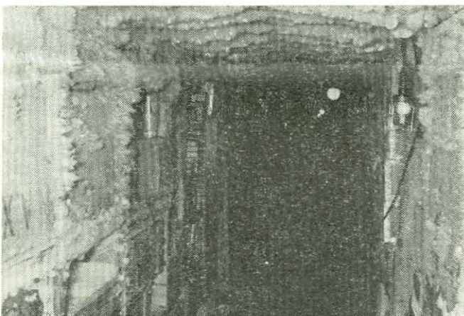
Fig. 1—Ice corridor, main building.
