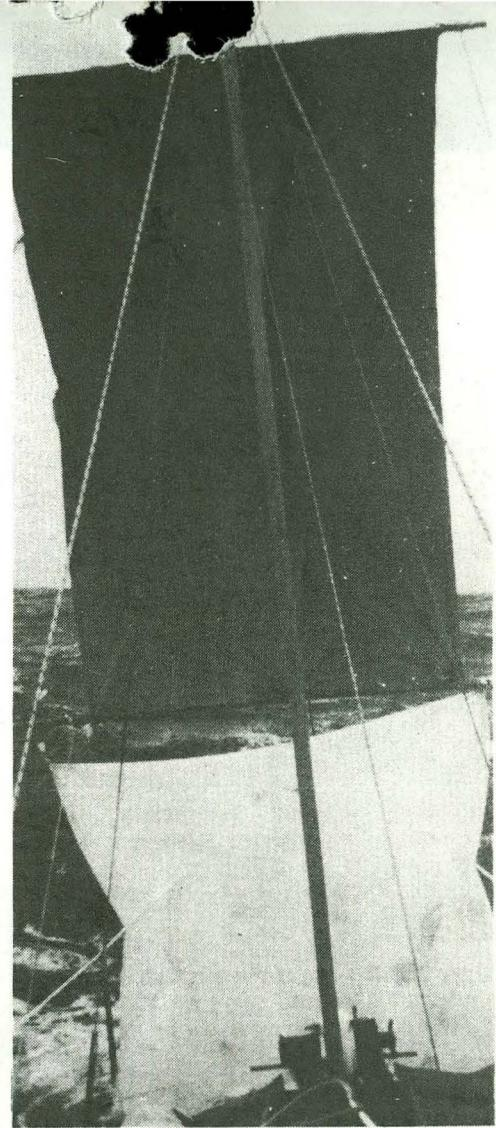
(ABOVE): For the first jury rig, on the way to Marion Island, a bed sheet was used as a lower sail. It lasted 700 miles before it blew out.
