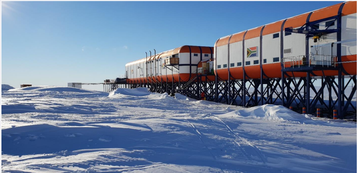
Figure 13: The research station's double story structure is built on stilts to avoid it being buried under snow. Notice the sastrugi (snow mounds) in front of the base. Block C can be seen in the middle of the picture, Block B on the right. Each block is 50 m in length. Photo: Camilla Kotzé.
