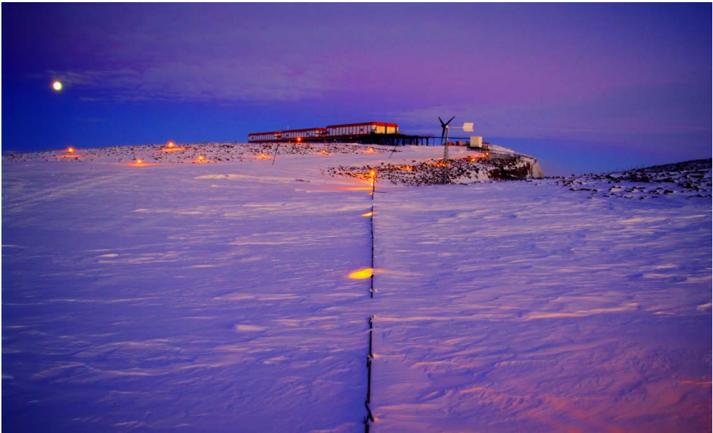
The diesel bunker and the fuel line between it and the base are well lit - this is essential for preventing mishaps during the times when it is necessary to refuel vehicles in low light or poor visibility conditions.
