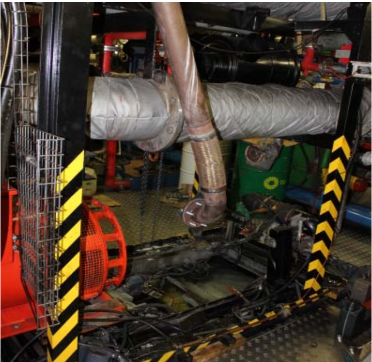
The genny room, with the empty frame of the generator (the alternator is the red unit on the left).
