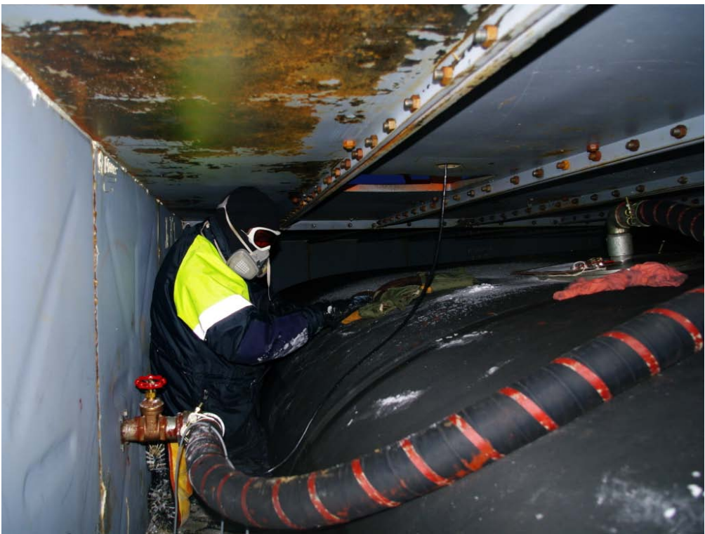
A peek inside the guts of the diesel bunker showing the enclosure and the 100 000 litre rubber bladder.
