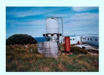
THE FIVE RESERVE WATER TANKS WHICH NEED A NEW STAND, TANKS SHOULD ALSO BE REPLACED,
