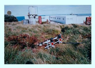
NEW FILTERS INSTALLED TO IMPROVE WATER PRESSURE ON HOT WATER CYLINDERS.
