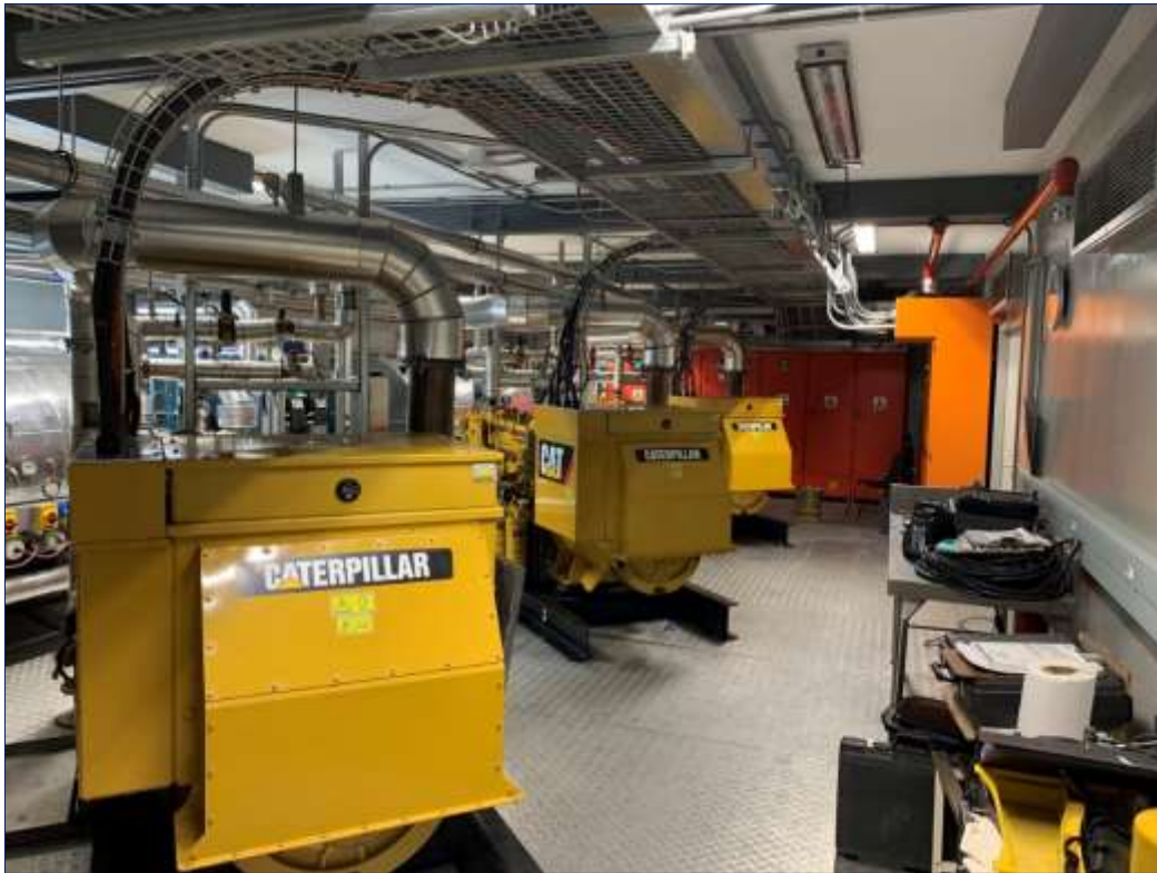
Figure 1. SANAE IV Generator Room with the 3 generators.
